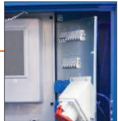
Swivelling installation plate with travel limitation
